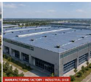
MANUFACTURING FACTORY / INDUSTRIAL SHED
