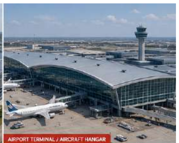
AIRPORT TERMINAL / AIRCRAFT HANGAR
