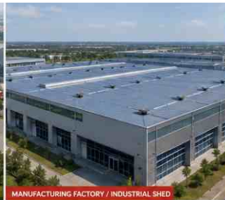
MANUFACTURING FACTORY / INDUSTRIAL SHED
