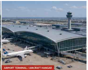
AIRPORT TERMINAL / AIRCRAFT HANGAR
